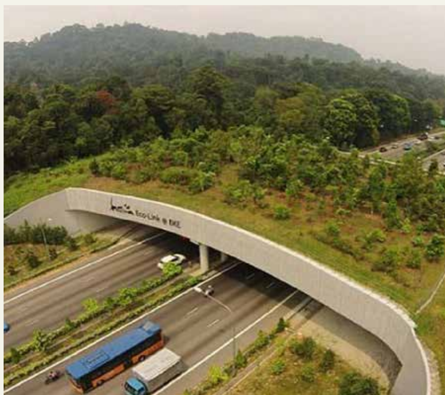
Figure 10: Animal overpass in Singapore built to protect animals from traffic
