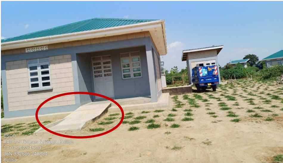
Figure 8: Ramp (in the encirclement) at one of the newly constructed RAP 2-5 Resettlement Houses in Ngwedo, Buliisa District.
